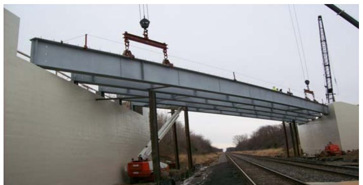
Setting girders atop new abutments.
