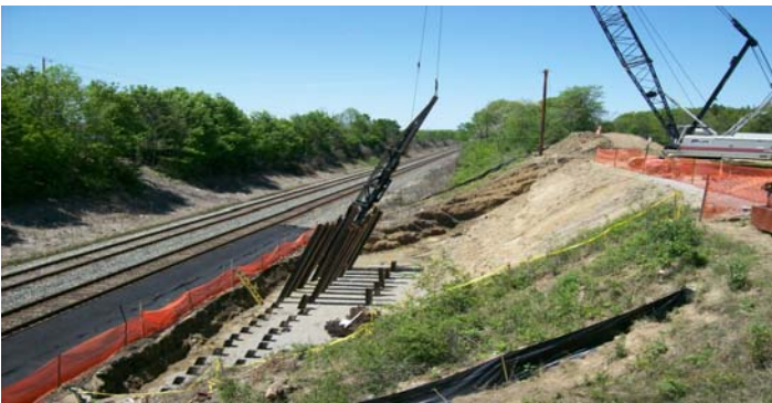
Quincy side pile foundations.
