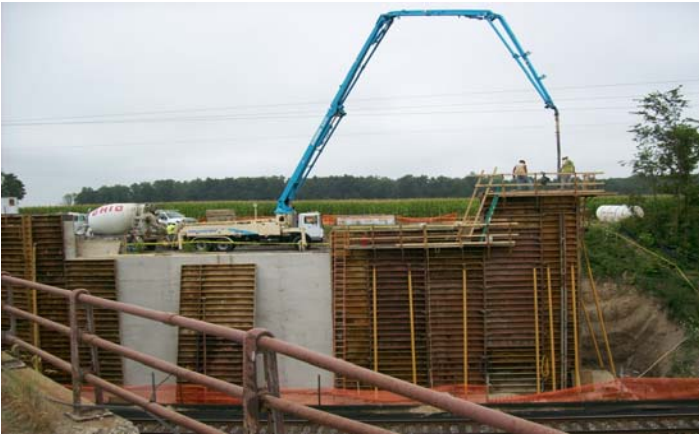
Pouring DeGraff side abutments.
