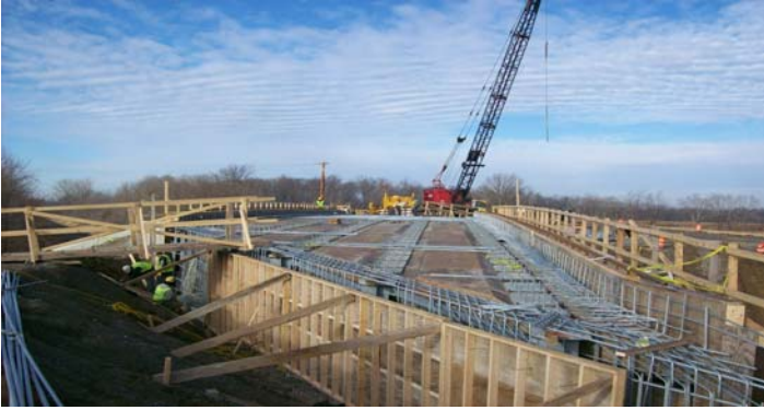
Rebar in place across the new bridge deck.
