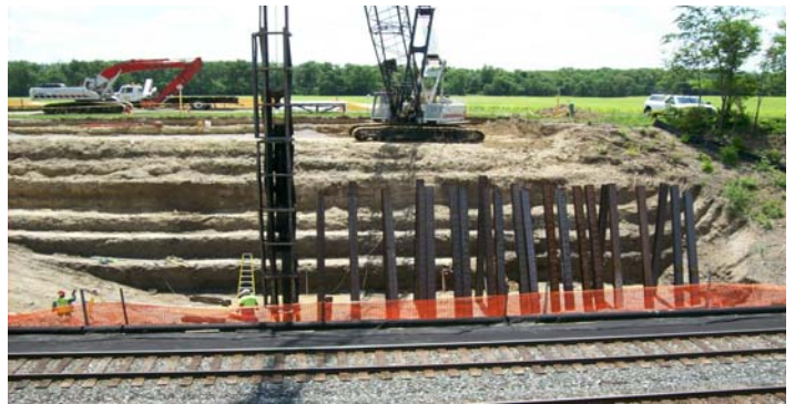
DeGraff side pile foundations.
