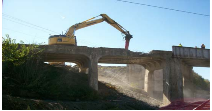
Demolition of 1925 bridge.
