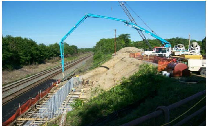
Pouring Quincy side foundation.
